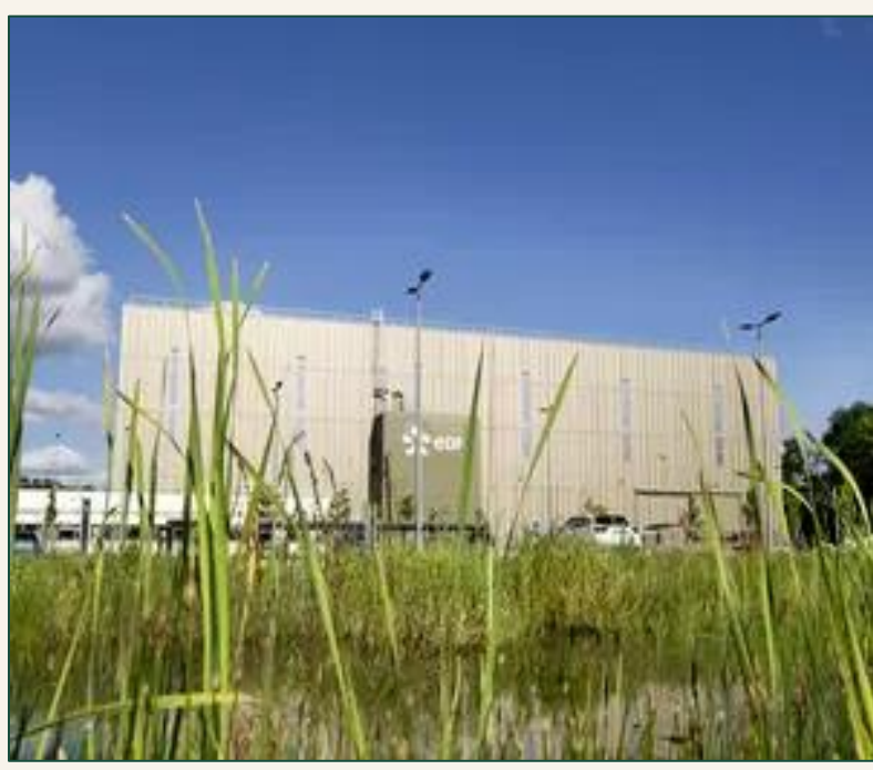
Graphite Reactor Decommissioning Demonstrator - France
